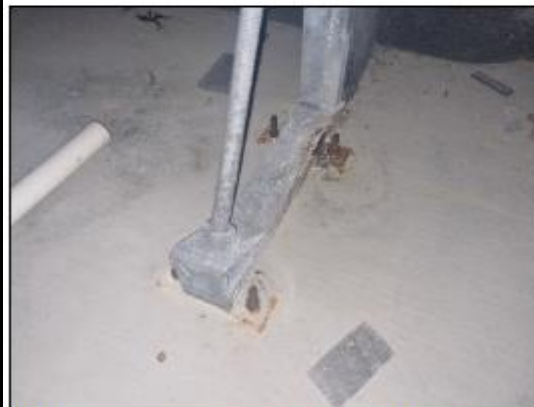
Photo 4 – Corrosion to base plates and bolted connections
