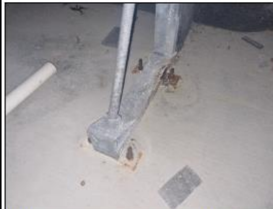
Photo 4 – Corrosion to base plates and bolted connections
